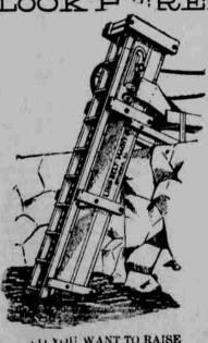
elevate from 300 gallons to 22,000 gallons per minute with the least possible power. It can be operated by windmill, steam, water or horse power.
