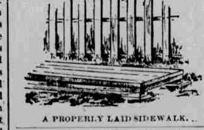
A PROPERLY LAID SIDEWALK.
