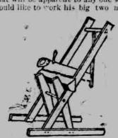
cross cut saw alone. The sawing arm into which the saw is inserted is slotted, as the saw will require freedom to slip up and down in the slot and is fastened by a pin through the cross slot .- Farm and home.
