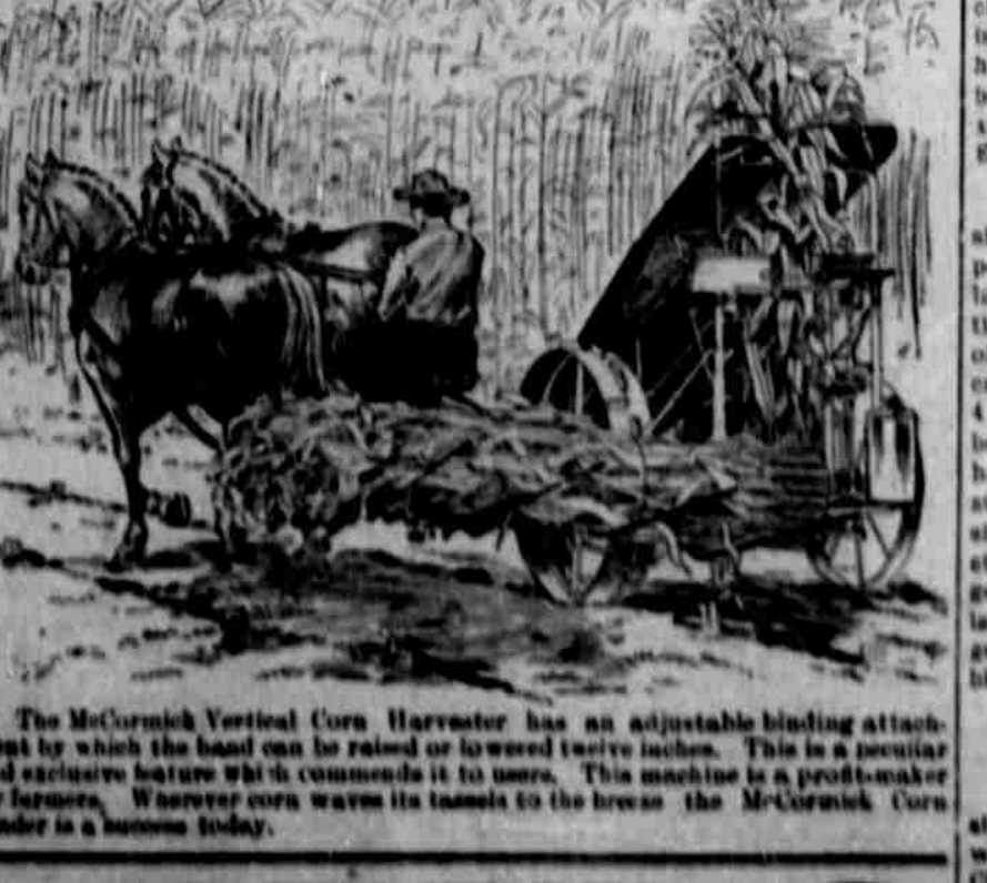
The McCormick Vertical Corn Harvester has an adjustable binding attachment by which the band can be raised or lowered twelve inches. This is a peculiar and exclusive feature which commands it to use. This machine is a profit-maker for farmers. Wherever corn waves its tassels to the breeze the McCormick Corn Harvester is a success today.
