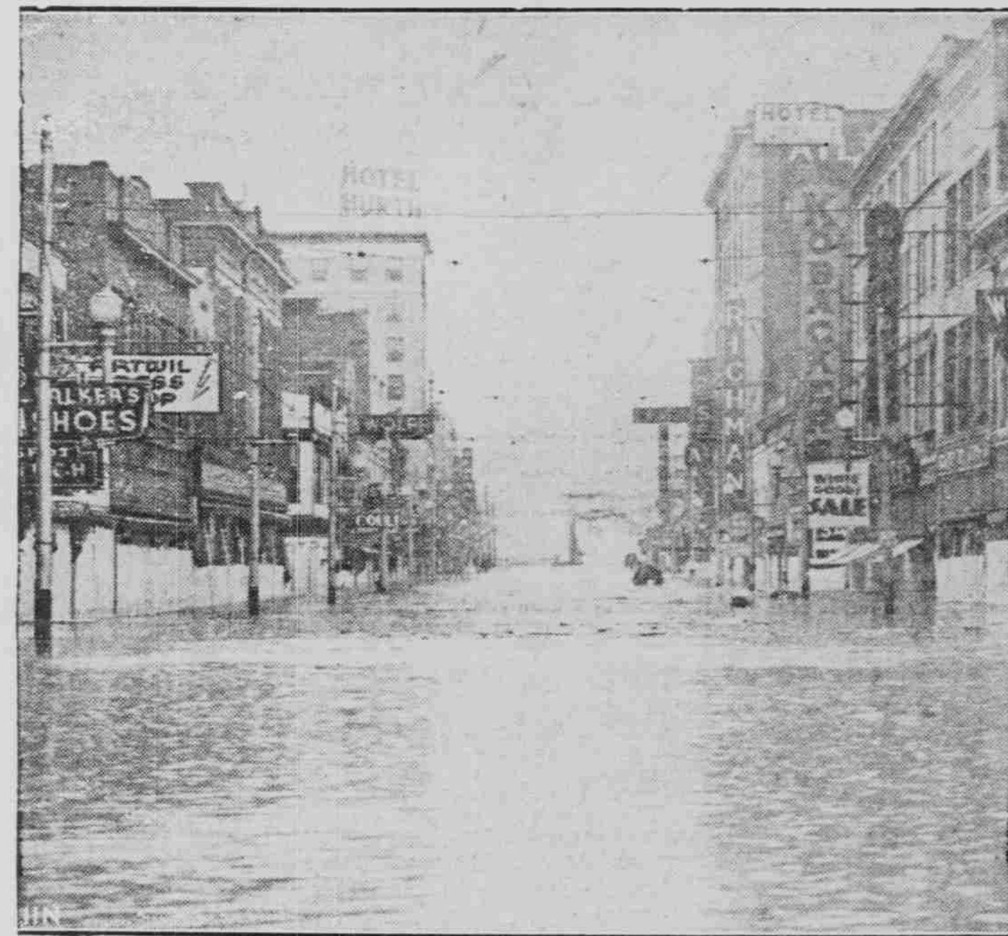
One might mistake this for a view of a canal, but it's Chillicothe street in Portsmouth, Ohio, where business was brought to a standstill and transportation paralyzed by the rampant Ohio river. Merchants protected their stores to an extent by boarding up their windows against the sweeping torrent. The flood has rendered thousands homeless.
