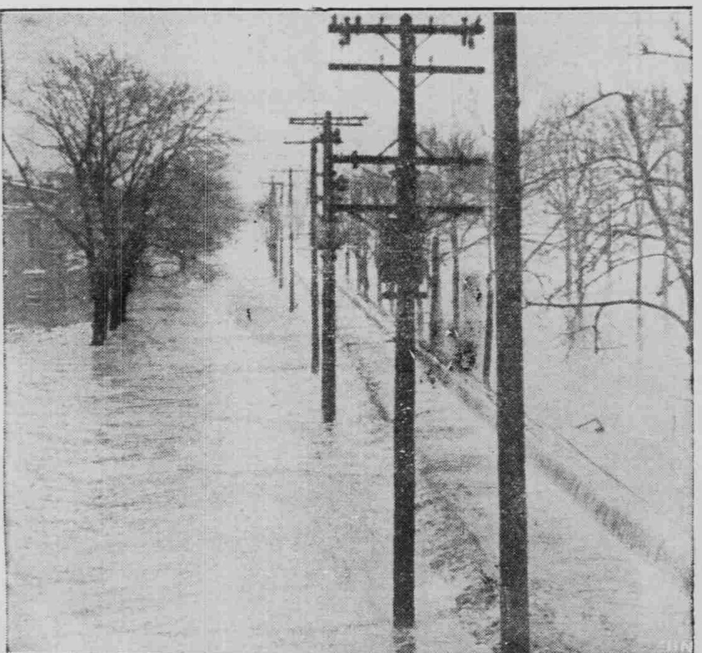
Some conception of the height of the flood that is raging in the Ohio valley is given by this graphic photo showing the surge of Ohio river floodwater over the dike at Portsmouth, Ohio, where thousands have been left homeless and property damage runs into millions of dollars. The river yesterday reached its highest level in more than 50 years.
