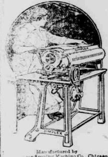
The Simplex is very simply constructed — its patent automaticfeed-boardcontrol makes possible a comfortable sitting position for the woman who irons. This saves health and strength! A life-time investment that pays for itself in a year. The Simplex is operated by electricity and heated by gas.
