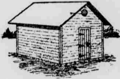
Exterior of Ice House.
