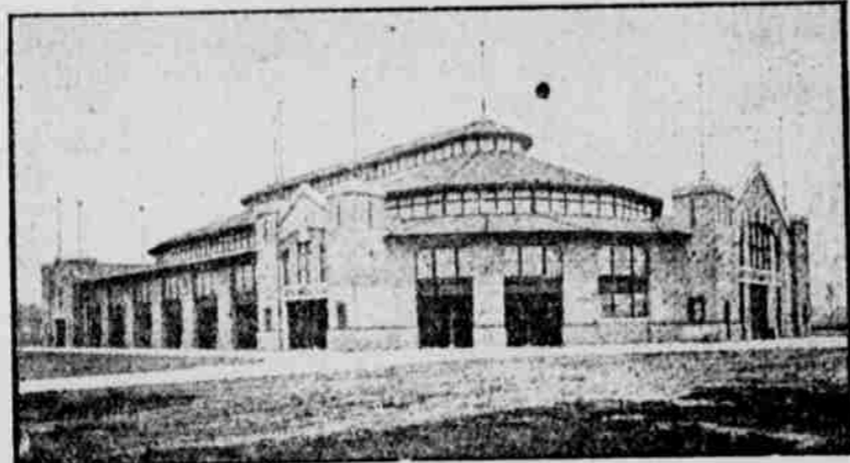
Stock Judging Building to Be Erected on Nebraska State Fair Grounds.
