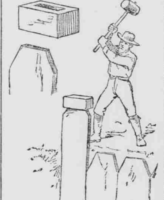
DEVICE FOR DRIVING PLANKS. A little wooden box or trough cut out of a solid piece of wood was placed at the top of the plank, as shown in the cut, and the mallet was pounded upon this.
