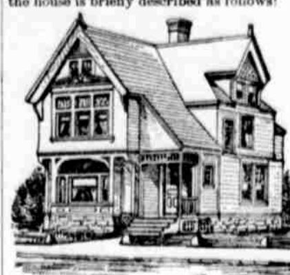
Stone or brick foundation. Height of stories—first, 10 feet; second, 9 feet 6 inches; cellar, 6 feet 6 inches.
