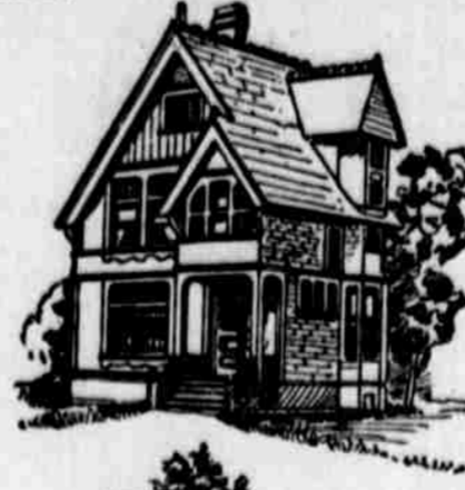
PERSPECTIVE VIEW. Frame Two Story Dwelling.—Height of stories—First, 9 feet 6 inches in the clear; second, 9 feet; cellar, 6 feet 6 inches. First story contains hall, 7x13 feet; sitting room (with fireplace, mantel and grate), 12x13;
