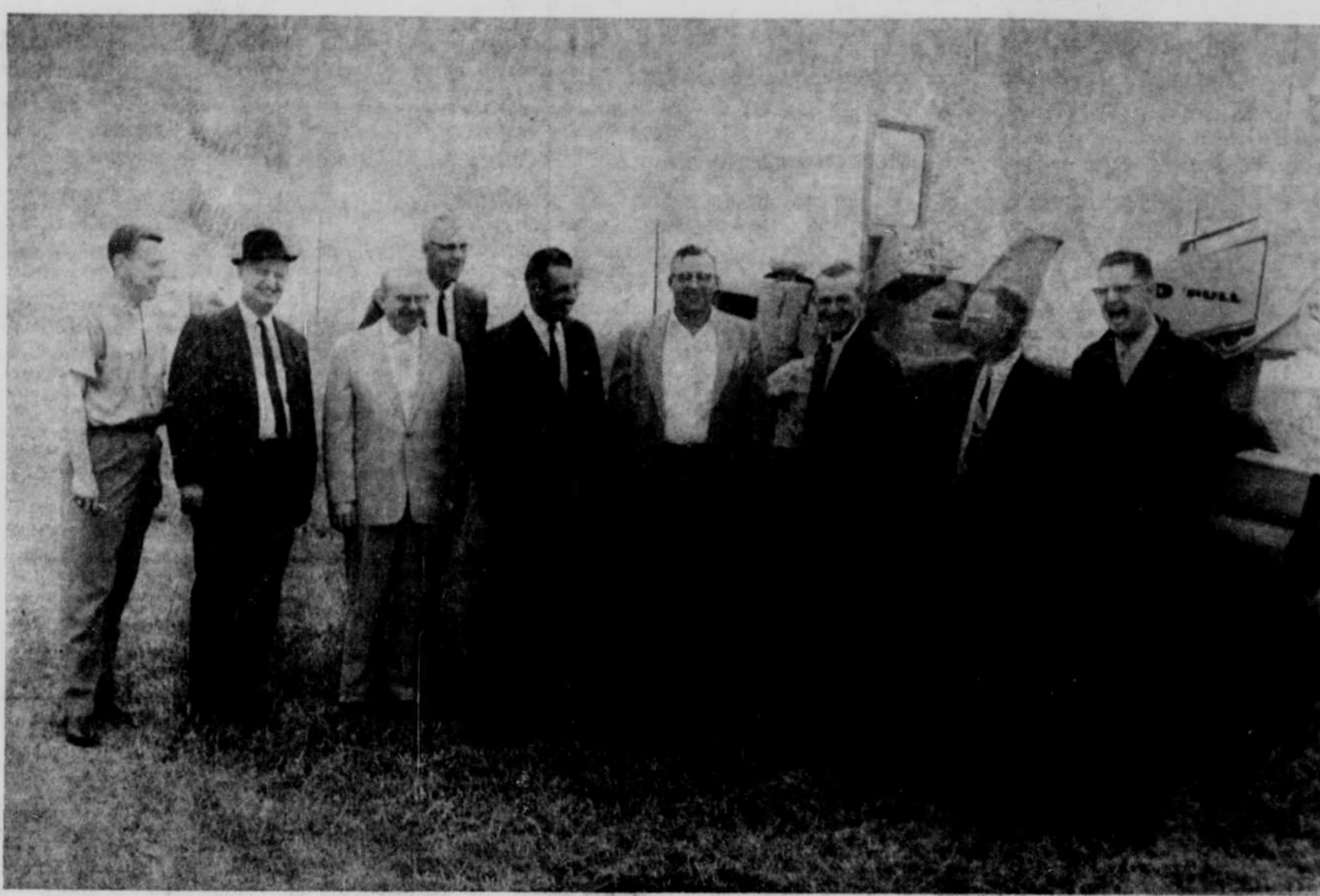
GROUND BREAKING CEREMONY — On hand for the turning of the first spadeful of dirt for the new Senior Citizens home were (left to right) Gil Poese, John R. Gallagher, Bill McIntosh, Judge Frank Cronk, Robert Golden, Howard Manson, Bill Griffin, Mr. Richardson and Kenny Curran.
