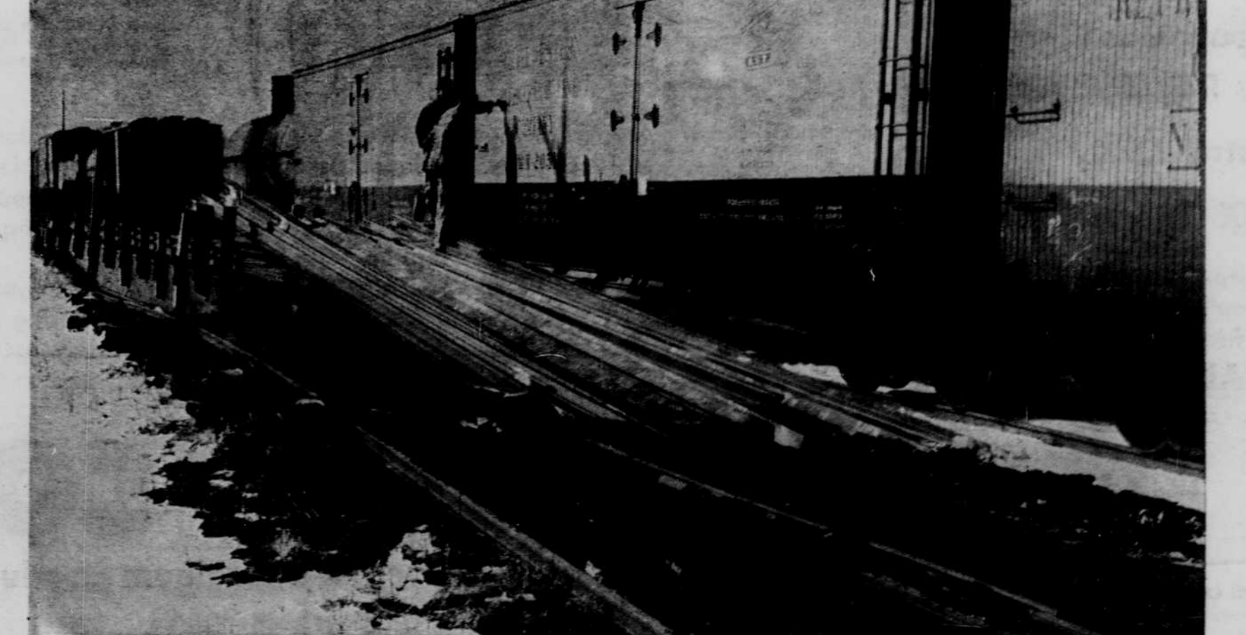
CHICAGO NORTHWESTERN tracks were torn up on both sides of the railroad crossing in O'Neill Wednesday when a locomotive and a flatcar loaded with rails jumped the track during a switching operation. The flatcar stopped on the west side of the crossing and the engine continued on over to the east side. Considerable track was torn up and the load of rails was spilled but no one was injured.
