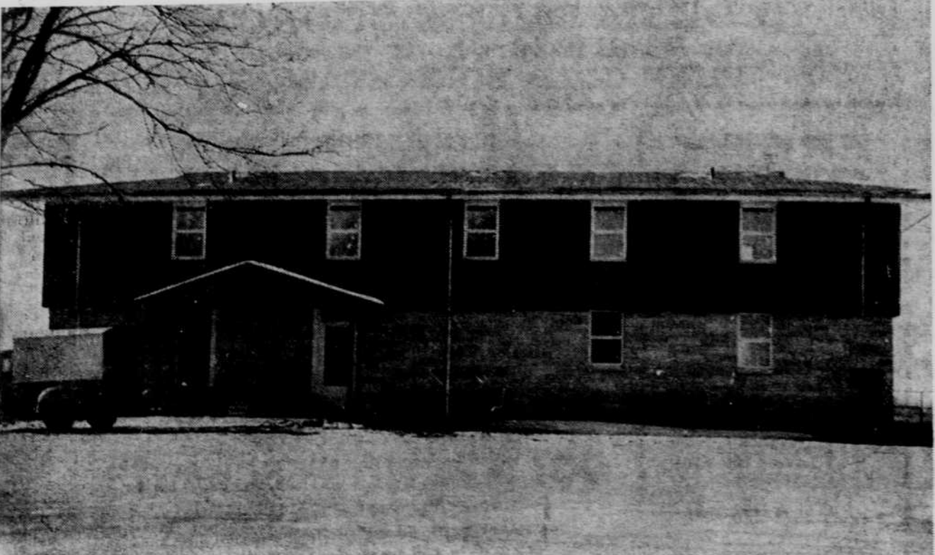
NEW ST. JOSEPH'S CONVENT — This new convent for the nine Sisters who teach in St. Joseph's school at Atkinson is in the final stages of construction. Interior finishing is expected to be completed about the first of February.
