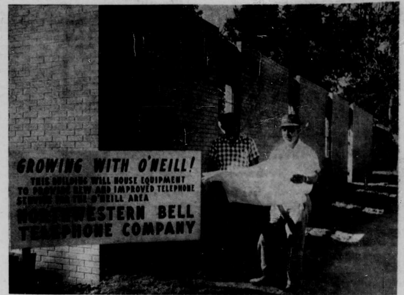
NORTHWESTERN BELL SERVICE supervisor Cash Arrasmith, left, is shown going over plans for the new telephone building here in O'Neill. Checking the plans with Arrasmith is Kurt Otte, of Otte Construction company, general contractors on the building. The new building, located at Fifth and Clay, will house dial equipment for the conversion slated for mid-1963.
