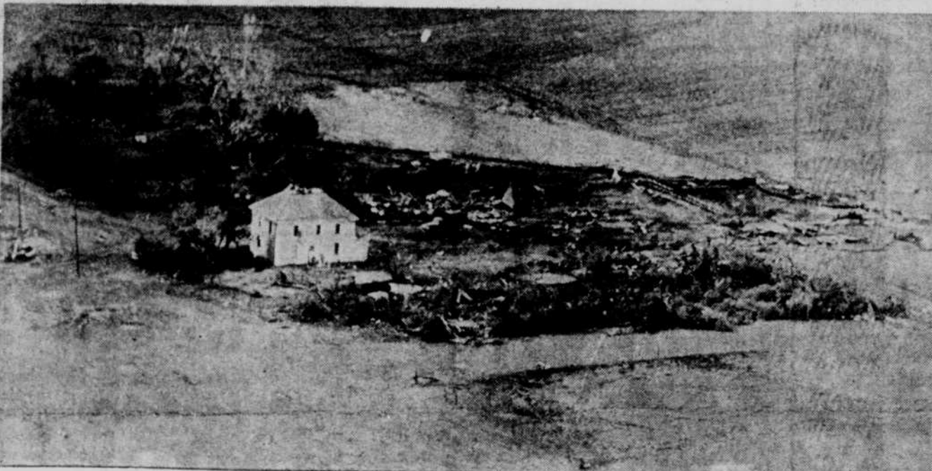
ONLY THE HOUSE REMAINED STANDING on the Jim Cerney place. Damage to livestock was light although some animals on the Lyle Kline farm were injured and had to be destroyed.
