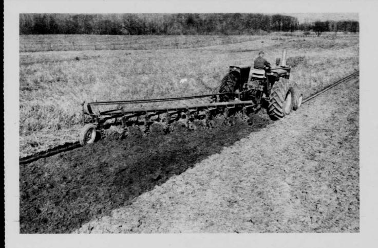
New, large-scale equipment is making it easier to wait until soil has the right moisture for good plowing. This eight-bottom, semi-mounted plow is new this year. It requires a near-90-horsepower tractor for power. These large mounted plows require somewhat different methods of adjustment than do pull-type plows. Be sure to check tractor tire pressure when using a mounted plow. Use the instruction manual for adjustments.
