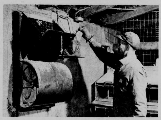
Here's a ventilation system that works well for this Indiana poultryman. When installing exhaust fans, always make certain they are in the wall away from prevailing winds. Otherwise, outside wind pressures will greatly reduce the efficiency of your ventilation system. Keep the fan motor dusted off and belts in proper adjustment. This can save you several dollars in needless repair bills.
