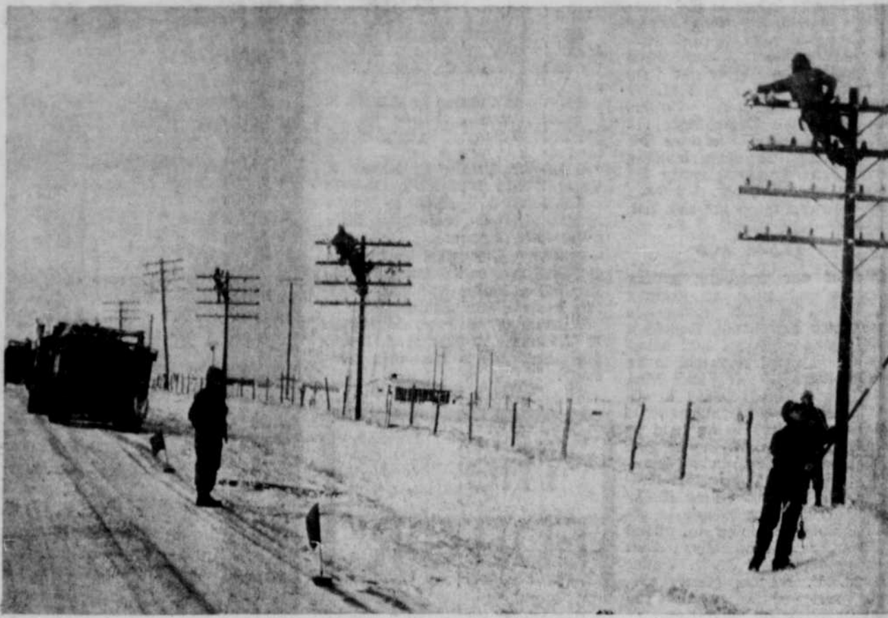
While some people were able to see beauty in the snow covered ground and sparkling ice-coated trees, workmen for the telephone and electric companies took a dim view of the whole thing. Bell Telephone repairmen are shown here repairing downed lines near the O'Neill Airport Tuesday morning. Some long-distance lines were in operation Wednesday east of O'Neill, but lines to the west were still out of commission. Lines in western Nebraska and South Dakota were hardest hit by the storm.
