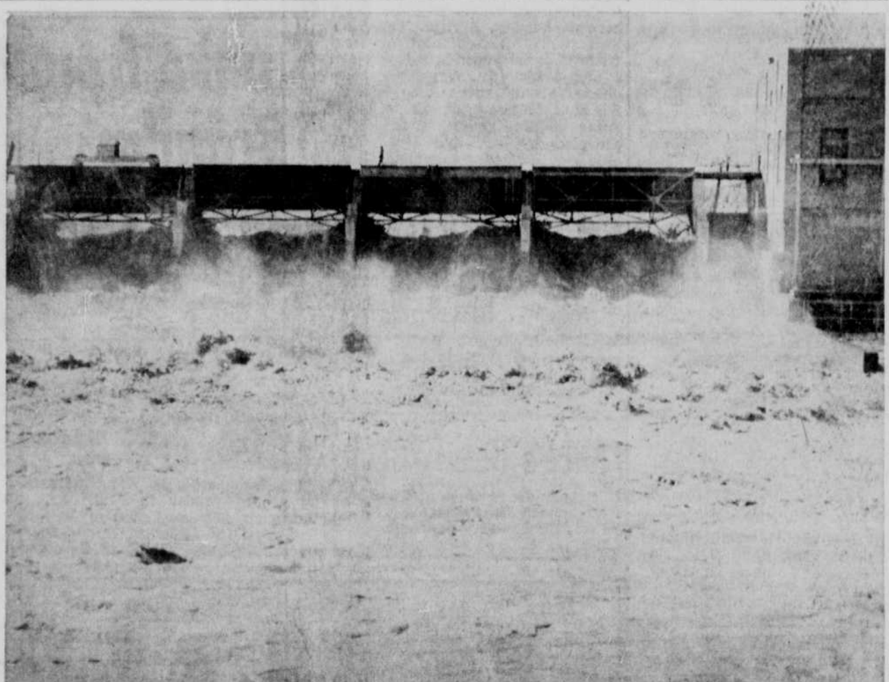
23,000 cubic feet of water was pouring over the Spencer dam Sunday as officials feared that the dam might collapse. All the gates were open and the flooding Niobrara river raced to its Missouri river mouth.
