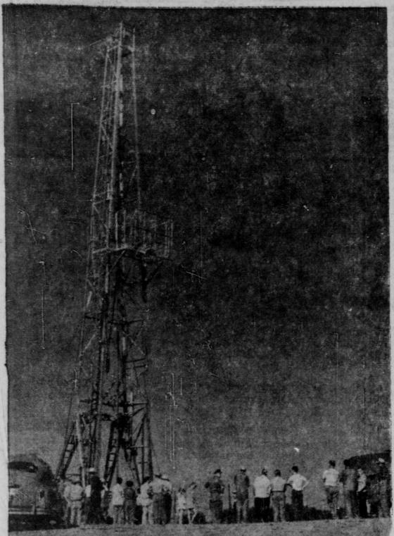
Test well on Neil Asher farm was going good until bit struck layer of granite at depth of 2,361 feet. - The Frontier Photo by John H. McCarville.
