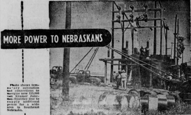
The connection of the new 115,000 volt transmission line to supply additional power and two-way feed for a large area in Southeastern Nebraska recently is symbolic of the extensive program now under way throughout Nebraska to bring more power and greater electrical benefits to Nebraskans.
