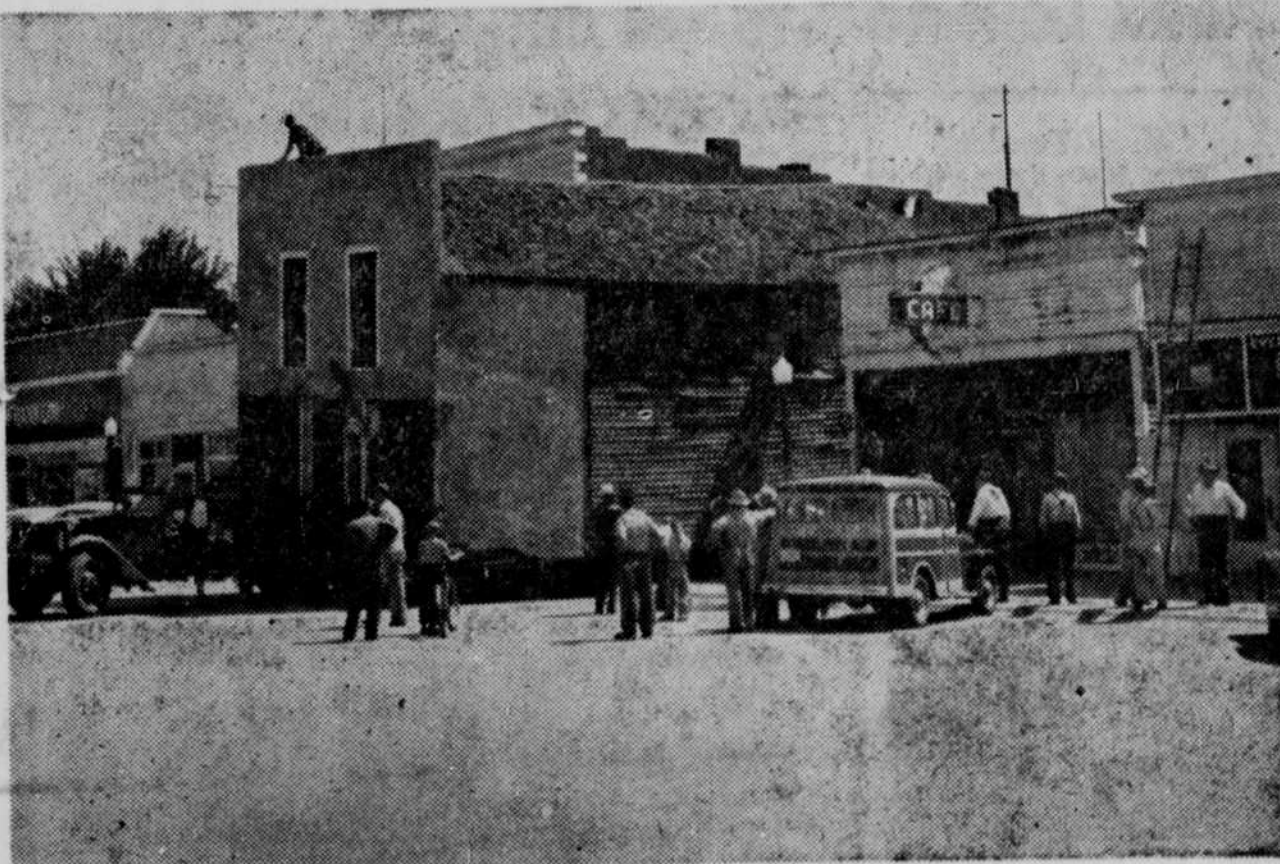
The former Harnish building, a frame 2-story structure owned since October, 1947, by Homer F. Mullen, was removed from the Douglas street scene on Thursday. New modernistic 2-story building will replace it (across from Golden hotel).—The Frontier Photo.
