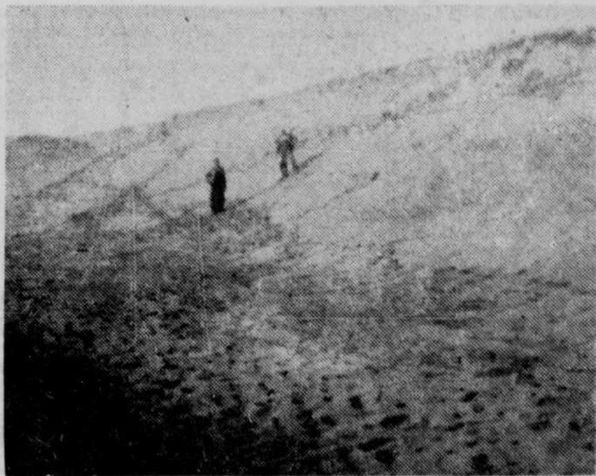
Harvey Tompkins (right) and Frank Musil, bulldozer operator and neighbor, are shown (above) surveying blowout area before sloping operations were begun. (Note tracks in loose sand). Bank is over 20 feet high, several hundred feet long. Location: One-half mile east and 3 miles south of Inman.
