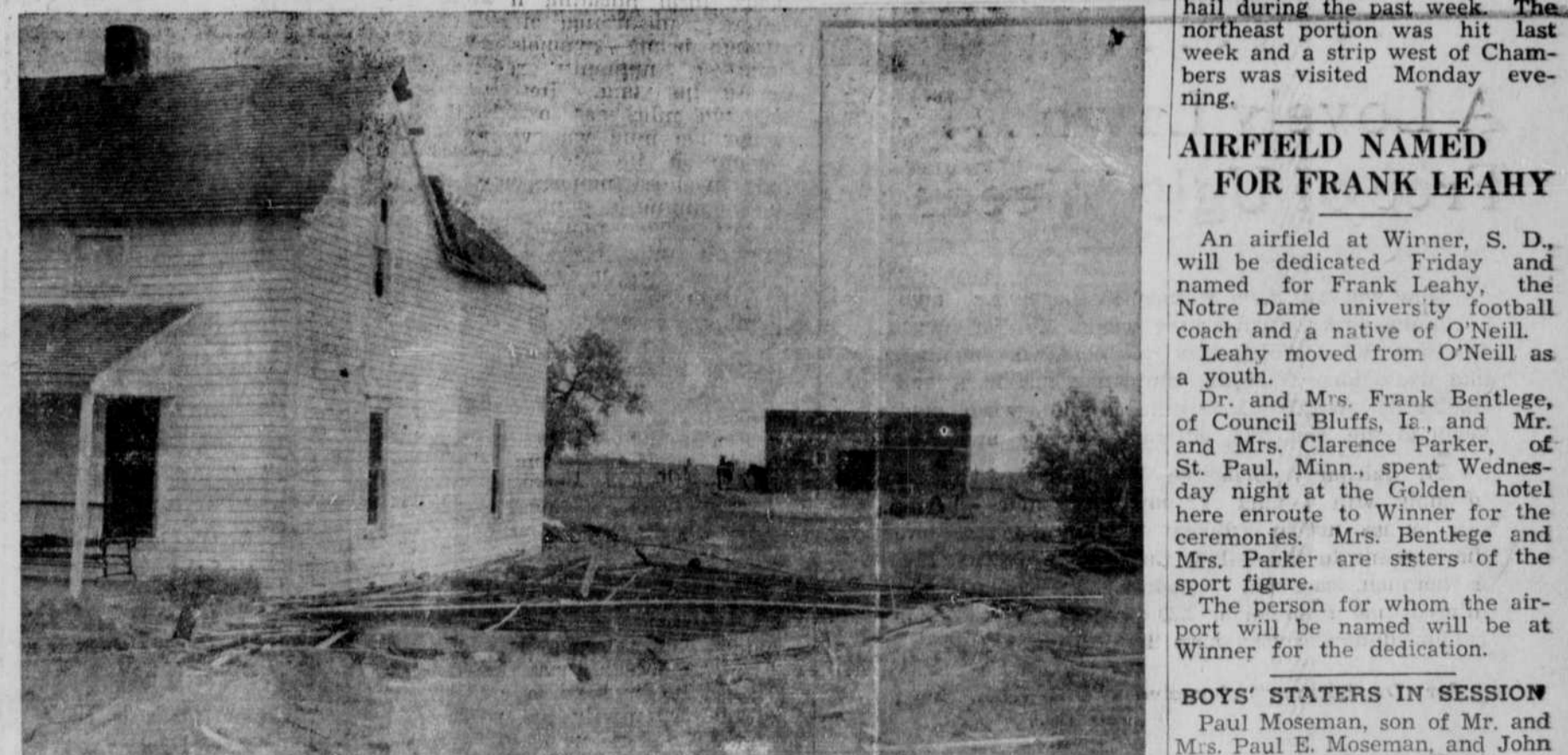
Probably the farm hardest hit by Monday's combination wind-hail-rain storm was the Fred Allen place, 3 1/2 miles southeast of Page. The roof was blown off the top of the barn (about 75 yards away) and a section of it lies beside the farm house. The upper photograph shows the west side of the house with splinter holes visible. The Allens are forced to abandon the house until repairs can be made. (See leading story on this page.)—The Frontier Photo by John H. McCarville.
