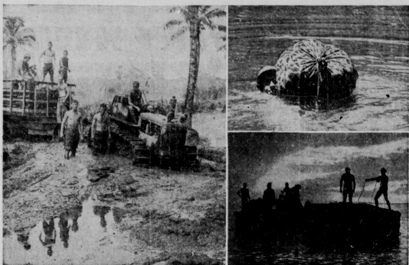
Left: Sandy mud plus daily rainstorms created this type of road for marines during their early days of operation on Bougainville. Jeeps and trucks were unable to get through to front lines until engineers and Seabees surfaced the roads with sea coral. Top right: Pfc. Juan Gonzalez starts across a lagoon in the South Pacific with an inflated poncho or rain cape. Bottom right: Marines work frantically against the setting sun. A whole day's work depended upon their success in getting a tractor raised before dark.
