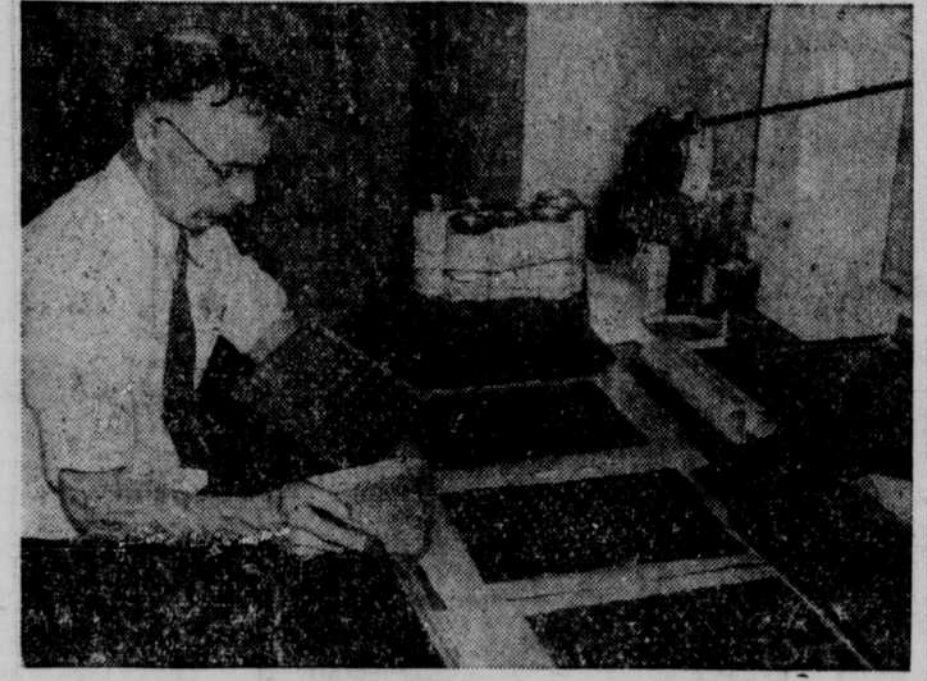
The vacuum counter which this man holds in his left hand automatically counts out the number of seeds desired for the "rolled-towel" germination test, and places them the right distances apart on a moist paper towel laid on a sheet of waxed paper.
