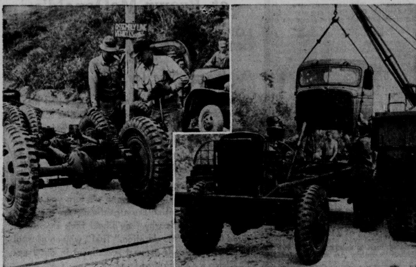
Mechanically minded American soldiers are taking their mass production assembly line methods with them to the Southwest Pacific. Here troops take parts of trucks, jeeps and ambulances as they come from the ships and put them through the line. One improvement on the assembly line system is their "Change over." When the boys tire of one operation, a command switches all members of the line to a new position and a new job. Left, rear running gear of a two-ton truck is assembled. Right, a cab is added to the truck and soon it will be ready for duty in a battle zone.
