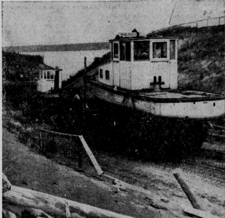
In transporting pipe and other supplies for a pipeline connecting the Norman oil fields of Canada with White Horse, on the Alaskan highway, to make fuel easily available for defense stations, U. S. army engineers overcome great obstacles. Here a convoy of supply barges and towing craft nears the end of a rough 16-mile cross-country voyage.
