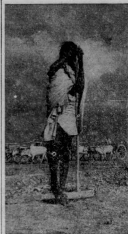
A picture out of an ancient world, primitive tools, bullock carts and hand labor, but all so necessary to the modern scheme of things, particularly war, for here is being constructed an airfield for American fighter, bomber and transport planes. A young girl laborer rests upon her crude tool. Broken stone, used to make a bed for the landing strip, is brought in by women who carry it in baskets upon their heads.
