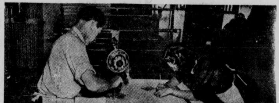
Layers of silk cloth are cut to specifications with a power knife.
