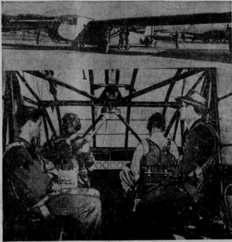
These pictures, just released by the army air forces, show the first of the new 15-place troop-carrying gliders, the CG-4A, now in quantity production. The glider can carry 15 fully equipped men, including pilot and co-pilot. It has a wing span of 83 feet, 8 inches, and a length of 48 feet, 3 inches. At the top we get a good idea of the glider's size by comparing it with the size of the men. Below is an interior view showing pilot and co-pilot at the controls.
