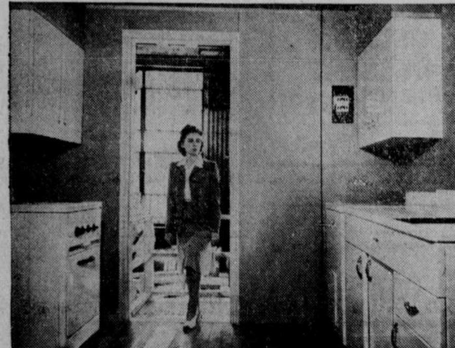
Everything but pork chops! A few hours after the first section of the "demountable" was put in place, milady enters the kitchen and finds it completely equipped and ready for business.
