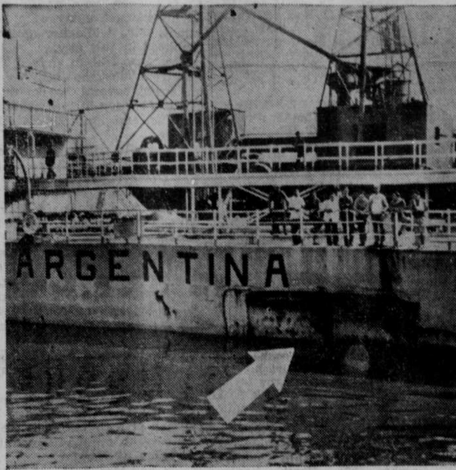
This view of the new 12,500-ton motorship Victoria, first ship under Argentine registry to be damaged by a submarine or a mine, shows the effect of the explosion. The Victoria was proceeding with her flag plainly visible, and showing lights at night. The ship continued to New York under difficult conditions, and managed to reach port safely.
