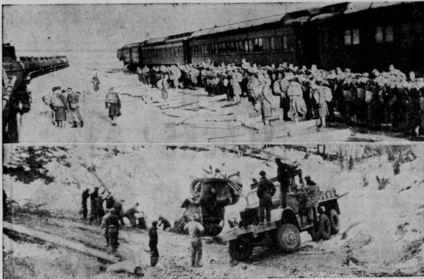
Upper picture shows journey's end, as U. S. engineer corps troops arrive at the end of the steel ribbon, at Dawson Creek, B. C., to start building a highway to Alaska from the end of the present road at Fort St. John. Below: First activity of road building at start of construction of the Alaska highway. Note men in foreground with truck pulling another road-building truck out of a ditch. All equipment for the project was shipped from the States.
