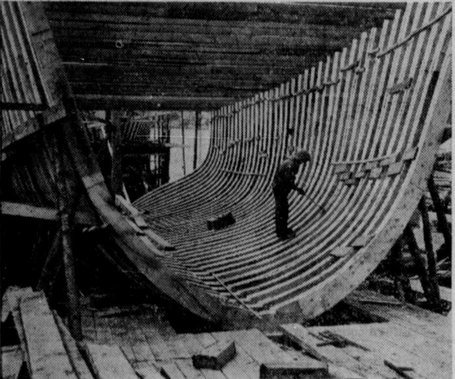
Old-timer Ray Rubshaw is working inside the framework of a hull under construction. He is dubbing or smoothing out and lining up the ribs for planking, using an adz.
