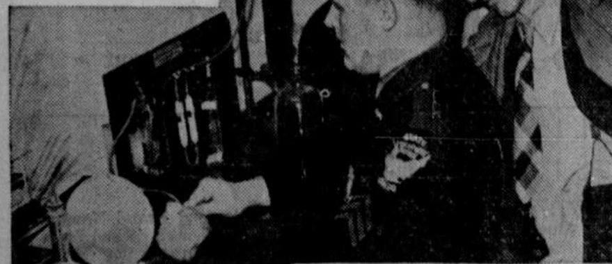
Test for drunkenness, which is made with a Harger drunkometer, a device which determines the amount of alcohol the driver has taken, from the air in his lungs.
