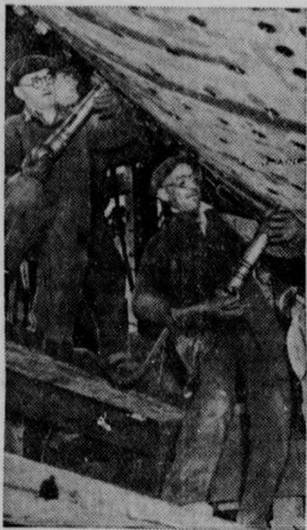
FINISHED PRODUCT—Plates, being designed in top photo, are being riveted to the bottom of the America in this picture. All plates are temporarily fitted together with bolts, which are being replaced here with the rivets, countersunk flush with plates to prevent resistance.
