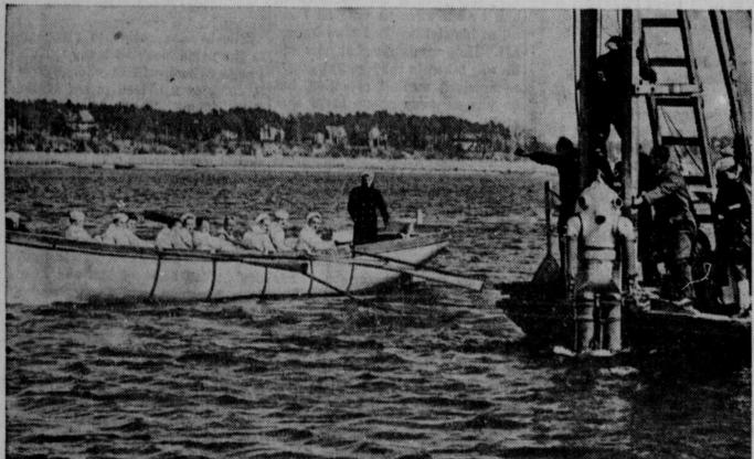
Cadets of the Admiral Farragut Naval academy watch as a new diving suit is tested in the Toms river to determine the feasibility of using a mixture of helium and oxygen for deep sea diving. The experiment was made by Cyril von Vaumann, traveler, writer and explorer. The diver controls the amount of air by manipulation of the valves of the tanks he carries with him. The suit weighs 1,100 pounds.
