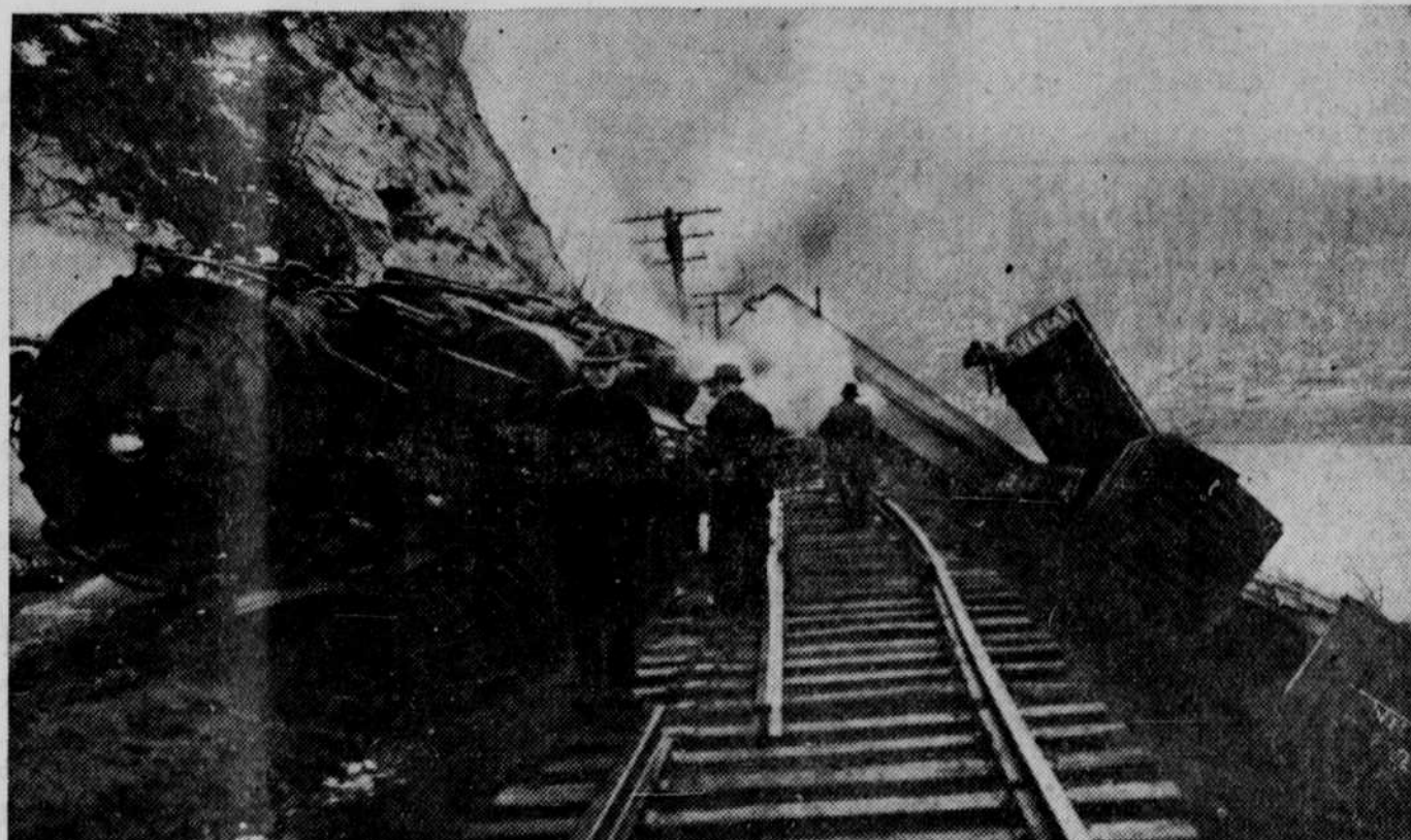
Rocks loosened by recent storms slid to the railroad tracks three miles north of Easton, Pa., causing this locomotive and 12 cars to crash down the embankment to the water's edge. Two of the cars were actually upended in the swollen Delaware river. The engineer and fireman were taken to a hospital.
