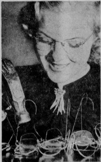
Miss Grace Fox demonstrates the durability of the new unbreakable eye-glass lenses developed by E. G. Lloyd of Beverly Hills, Calif., as she uses a hammer in trying to break them.
