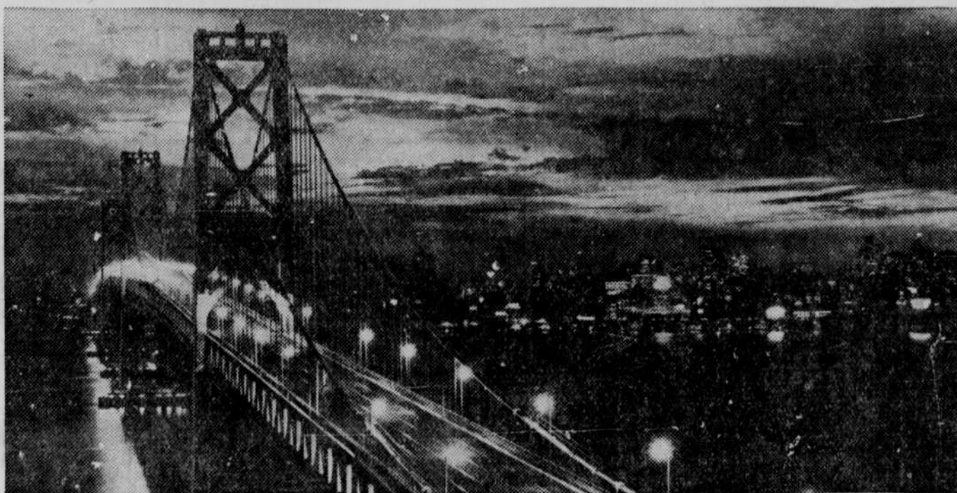
The world's largest sodium lighting installation, the first completed section of the Golden Gate bridge to Oakland, looking toward San Francisco from Yerba Buena island. Nine hundred and twenty-four sodium lights, the equivalent of 35 full moons makes the highway so bright that car headlights are unnecessary.
