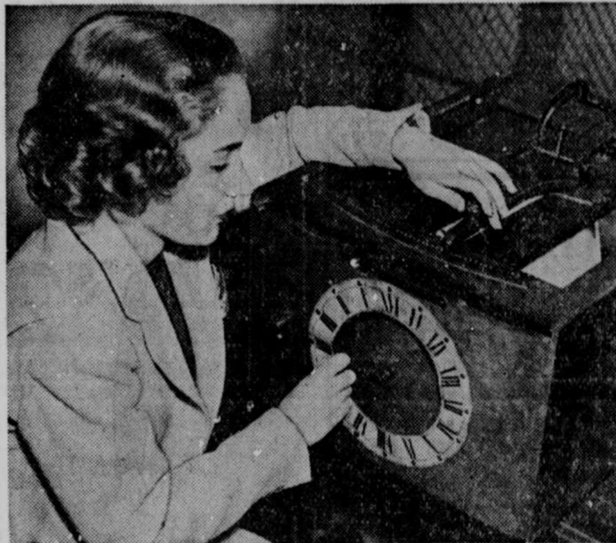
Photo shows Miss Lorraine Vocco, of New York city, demonstrating the model of the first United States typewriter now on exhibition at the Smithsonian institution. It was invented by William Austin Burt in 1829. The crude wooden machine was never produced commercially.
