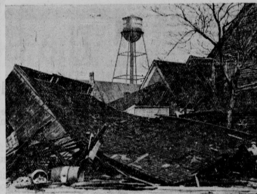
Two lives were lost and much property damaged by a wind storm which swept the city of Detroit. The photograph shows a large barn wrecked by the sixty-mile gale.
