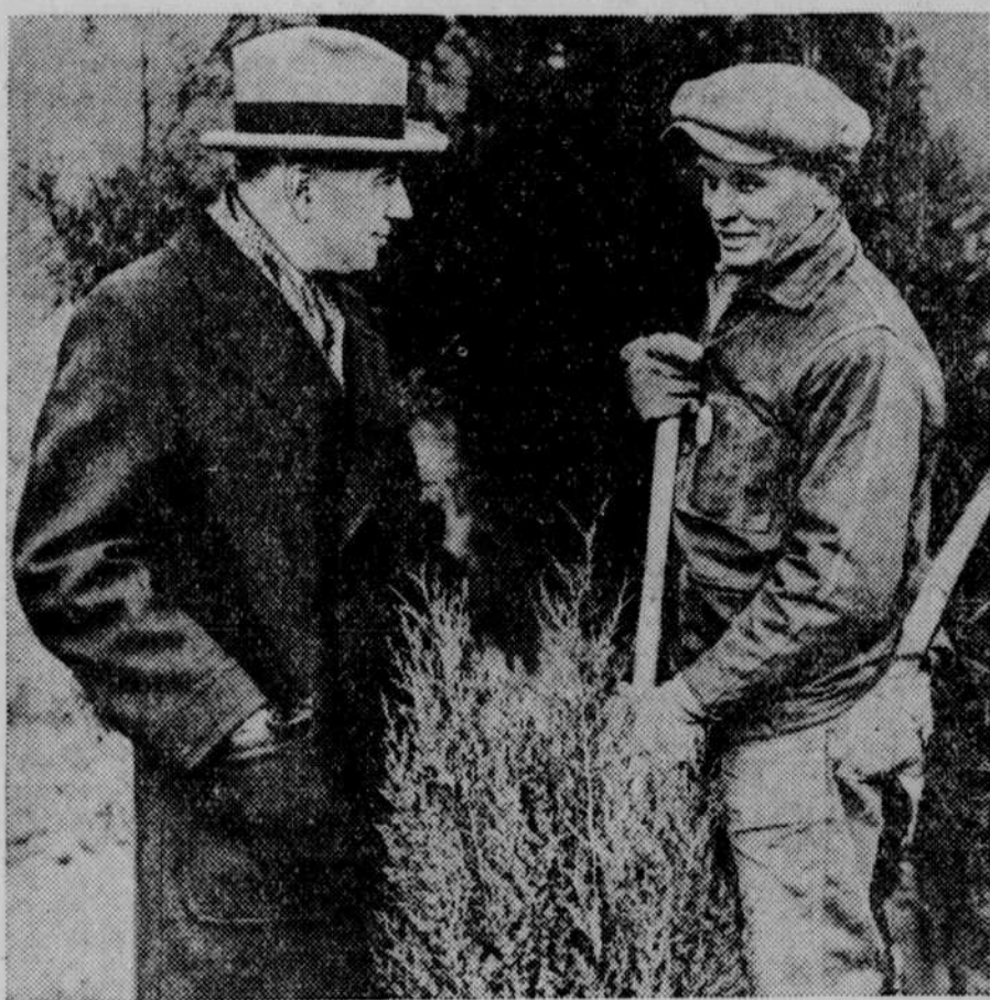
Rex Tugwell, undersecretary of the Department of Agriculture, is talking to Jesse Trimble, PWA worker, during Rex's visit to "Tugwelltown," a new building project at Berwyn, Md.
