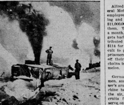
F OUR rotary snow plows were at work on Cumbres Pass, Colo., 10,015 feet above sea level, clearing the way for three Denver and Rio Grande long youth-rather than prolong Western trains barricaded by immense snow drifts. Eighteen passengers were marooned in the cars. High biting winds, icy tracks, steep grades, not mean childhood, but the years all made it exceptionally difficult to clear the way. It took 72 hours to
