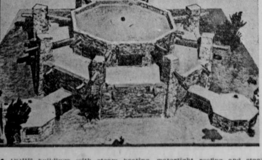
ADOBE buildings with steam heating, watertight roofing and steel window frames in the modern manner will be features of the new capital on the Navajo Indian reservation in Arizona. The building of the Navajo capital is being financed by a Public Works administration allotment of $500,000. The photograph shows what one of the dwelling units will look like when finished.
