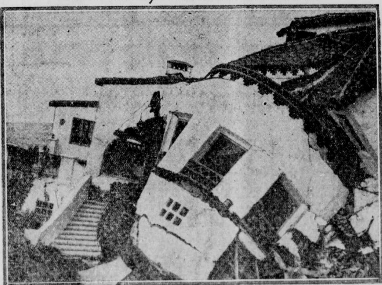
Following the collapse of a 200-foot cliff at San Clemente, Cal., the beautiful $50,000 mansion of Mayor Thomas Murphine is reduced to the mass of cracked masonry and twisted wreckage shown here. The landslide also blocked the main line of the Santa Fe railroad.
