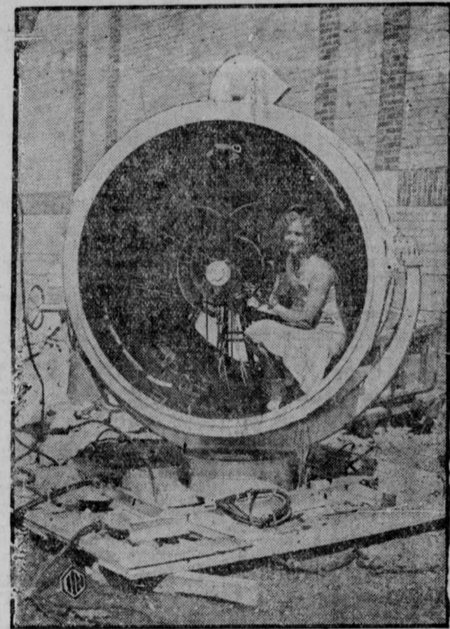
The Lindbergh Beacon Light, just before it was hoisted atop of the Palmolive Building, Chicago, 620 feet above the street. It is similar to those used in the fortifications on the Panama Canal, and is equivalent to a half-inch section of the sun, being two-billion candle power. Airplanes flying at an altitude of 43,000 feet can see the light at a distance of 250 miles. (International Newsreel)
