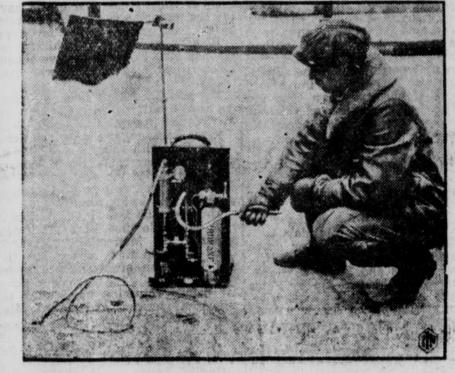
Testing the manhole gas detector developed by George W. Jones, explosive chemist for the United States Bureau of Mines at Pittsburgh, Pa., for use in city streets. It is believed that by placing watchmen on the streets in order to sample the air in manhole entrances, it will be pessible to considerably reduce the number of serious explosions from escaping par.
